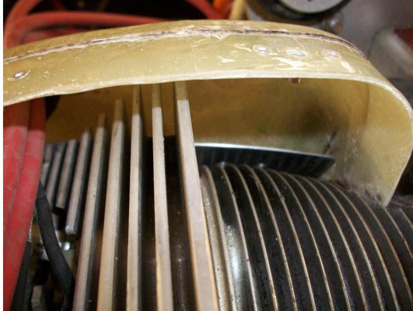
Figure 21. In the picture above, even the aft end of the duct was tightly sealed to assure all the air exited the plenum between the cylinder fins only.
