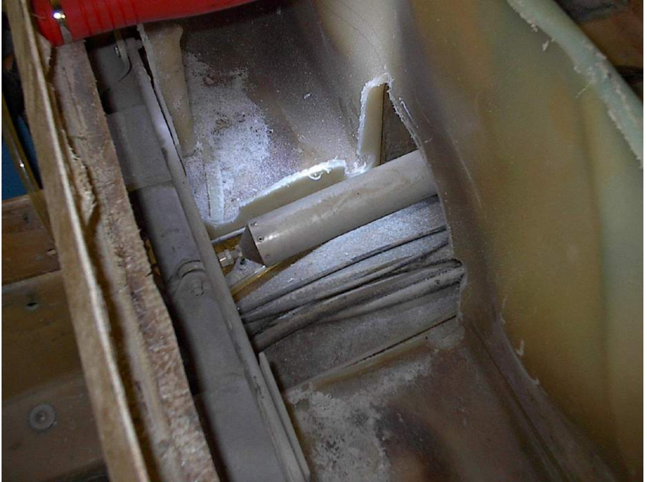
Figure 6 Carefully cutting around the controls.
