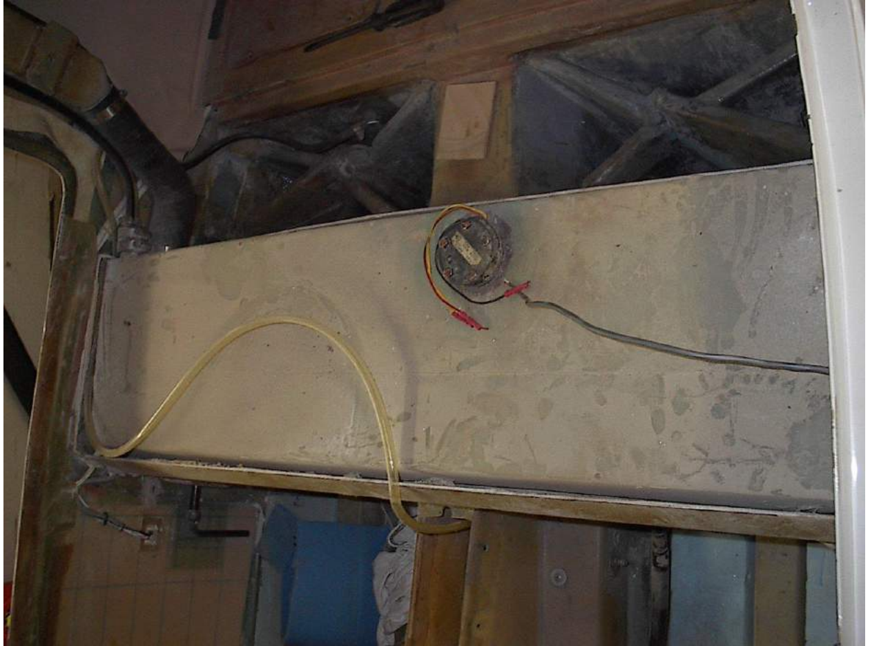
Figure 4 Tank top now exposed
